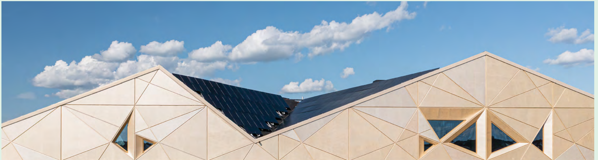
The Juvelen building in Uppsala, Sweden (Viedoc's headquarters)
